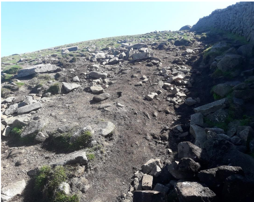
Figure 6.1: A heavily eroded section of path on Slieve Donard illustrating the fragility of the shallow, friable soils under pressure from increased foot traffic and more frequent heavy rain events. Image taken August 2021.
