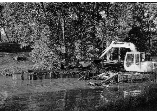
The floating dredger at work.
