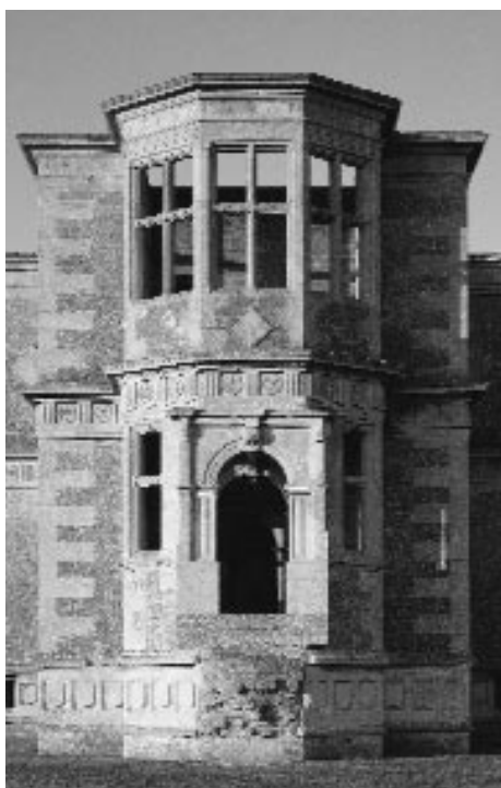
The North Wing and front door in the early morning. Begun by Sir Thomas Tresham in 1594, the lodge is now a roofless shell in the form of a cross with interesting friezework.
