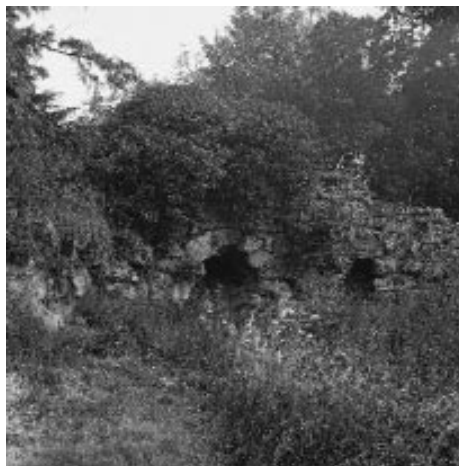
View of the Grotto surrounded by undergrowth and weeds.
