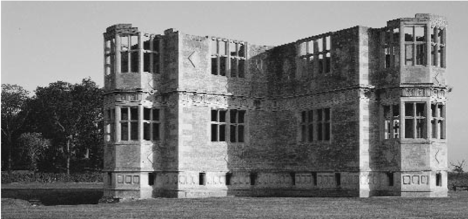
A view of Lyveden New Bield, taken from the south-east showing the south and east wings.
