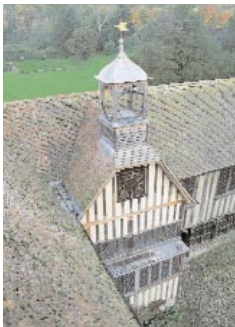
Ightham Mote, interior courtyard, looking northwards.
