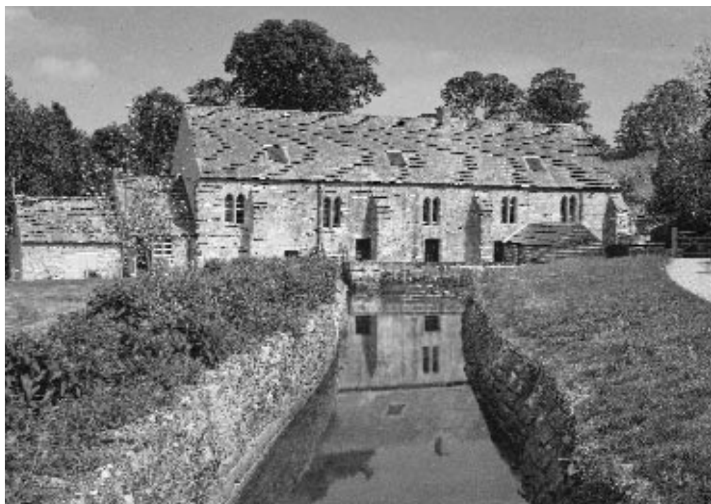
Fountains Mill the finest surviving example of a monastic water mill 800 years old. West front showing mill race.
