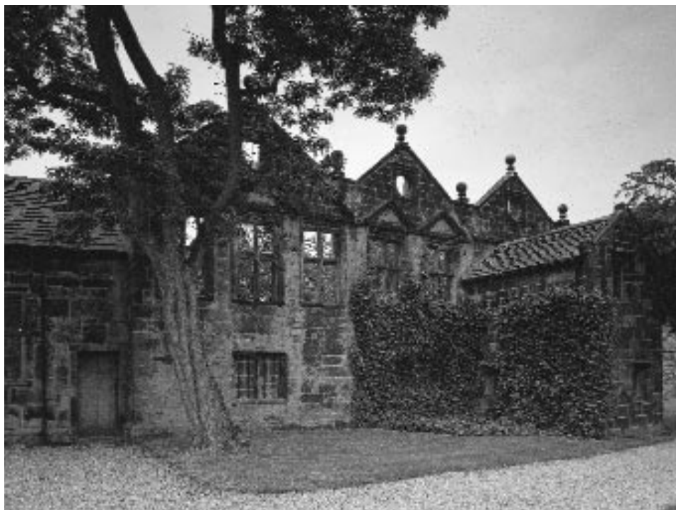
East Riddlesden Hall, Starkie Wing. Only the exterior wall is left standing
