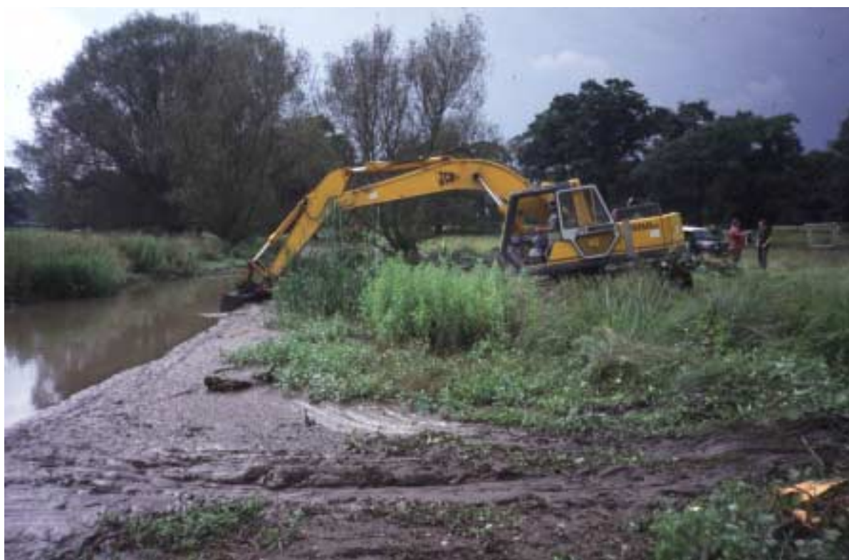
Dredging in progress at Kedleston. Simon Hiley.
