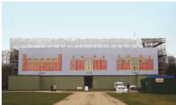
Roof restorations underway at Dunham Massey
