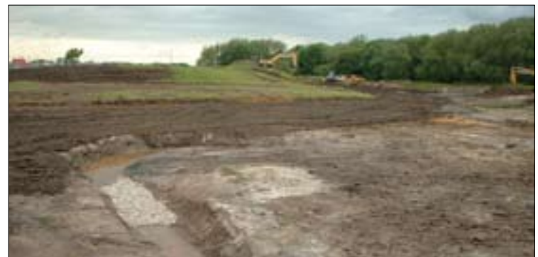
The newly constructed channel
