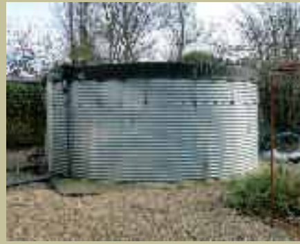
Rainwater collection tanks at Nymans in Sussex harvest enough rainwater to last the whole summer
