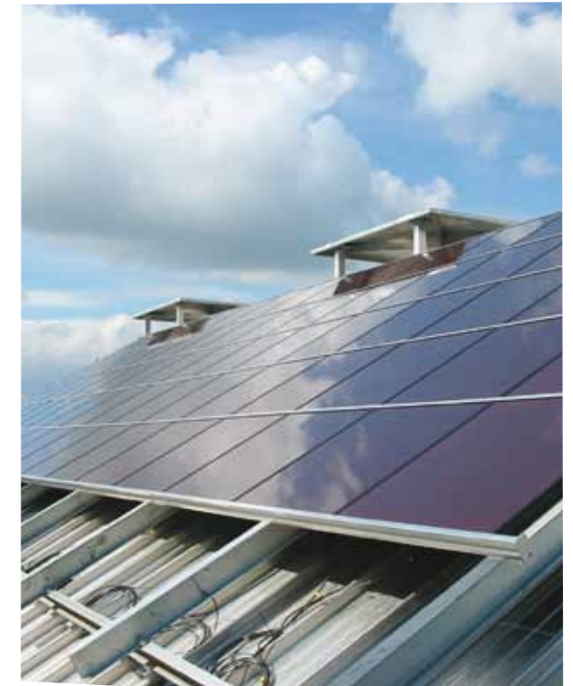
Our central office in Swindon (above) is home to our largest solar electricity installation, with 1554 PV panels. In 2008 the panels generated 80 MWh electricity – providing around 30% of the building's electricity needs and exporting to the national electricity grid when office demand is low.
