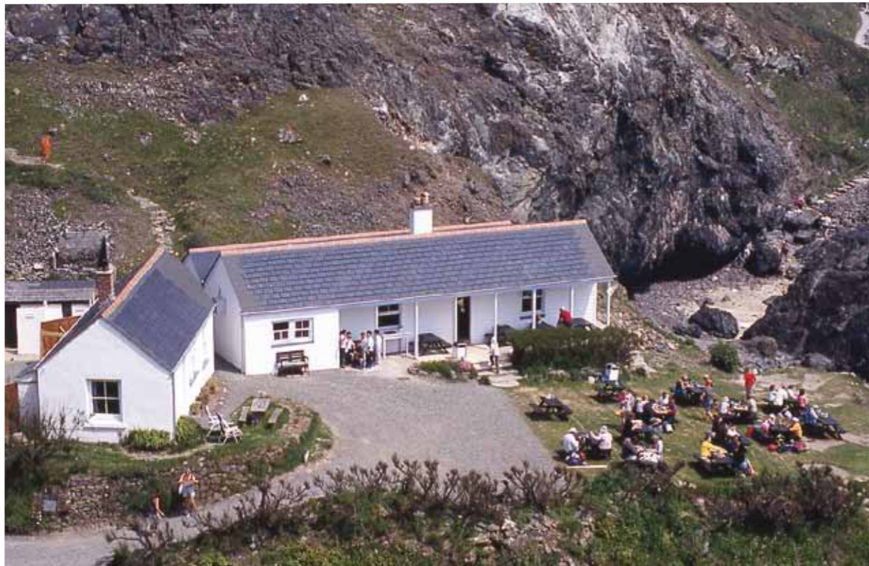
The solar slate panels on Kynance Café, Cornwall, are designed to look like conventional slates. The roof makes all the electricity needed and blends in with the coastal landscape. The café was the second place in the UK to use this innovative solar slate technology.
