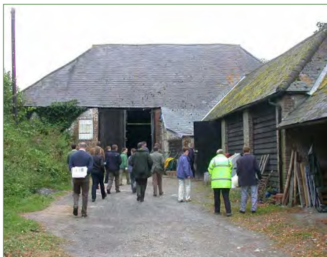
Barn, Saddlescombe Farm, Sussex: Adaptive Re-Use training day
