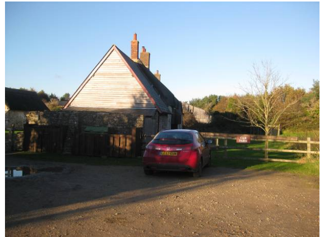
Car park area
