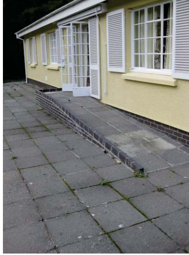
Ramp from sitting room to patio
