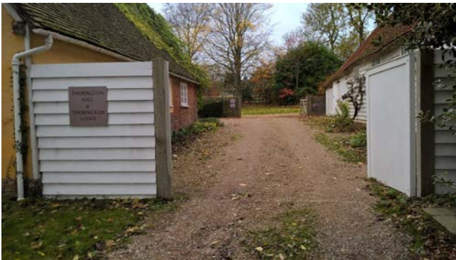
Outer entrance gates to gravel drive
