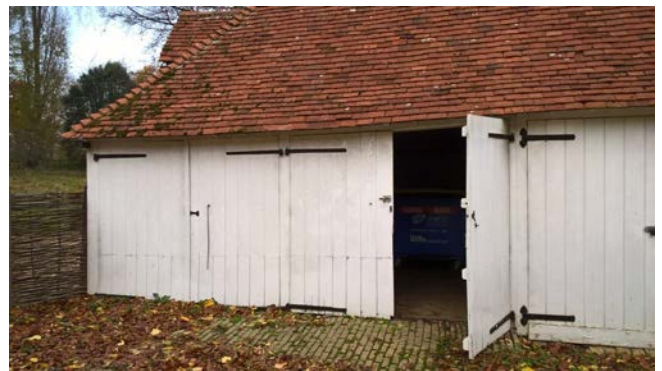
Outbuilding for refuse storage
