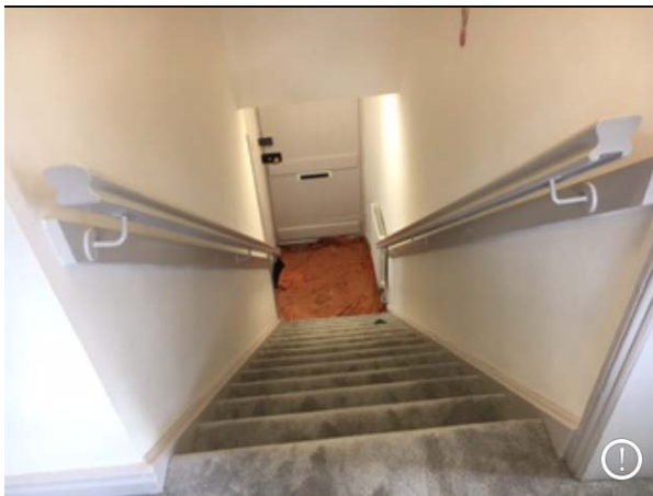
Staircase and handrails (protective cover at door)
