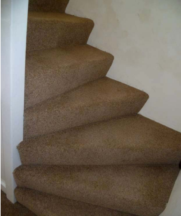
Staircase to first floor
