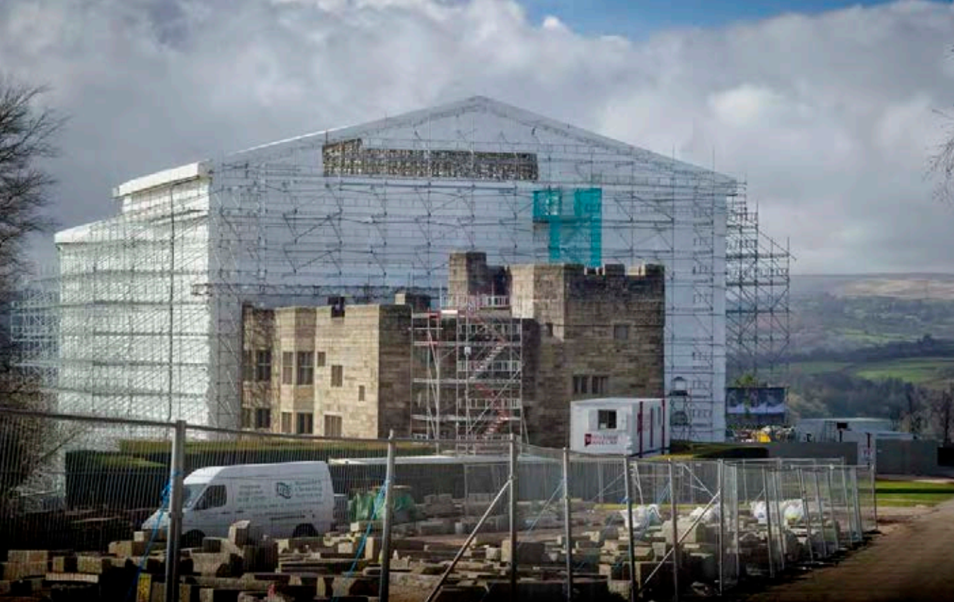
1. Castle Drogo under its vast scaffolding canopy All photos: National Trust/Tim Cambourne
