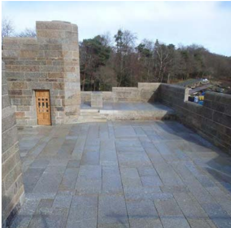
3. Paving on the north roof: the re-roofing project presented an opportunity to reinstate the original granite slab finish
