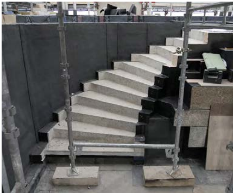
4. The North Tower stairs, showing the complex detailing of the membrane and damp-proof course
