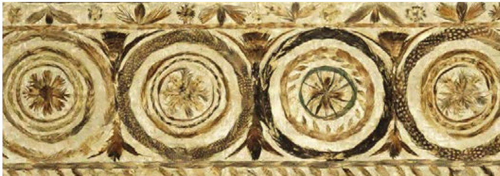
3. Detail of the feather frieze in the Drawing Room: the pattern is formed from hand-cut poultry and game-bird feathers fixed in place with isinglass
