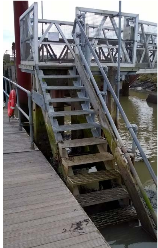
Steps from the pontoon at mid-tide
