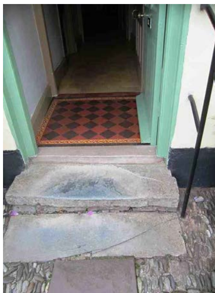
Steps up to the front door
