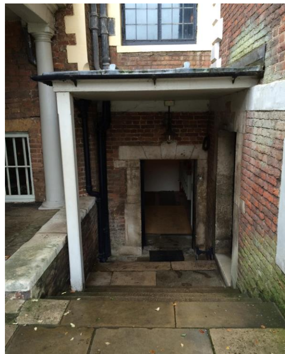
Entrance to basement via steps
