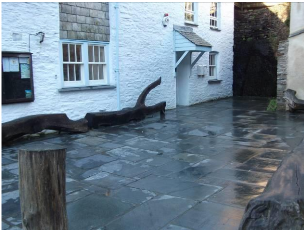
Courtyard leading to main entrance door
